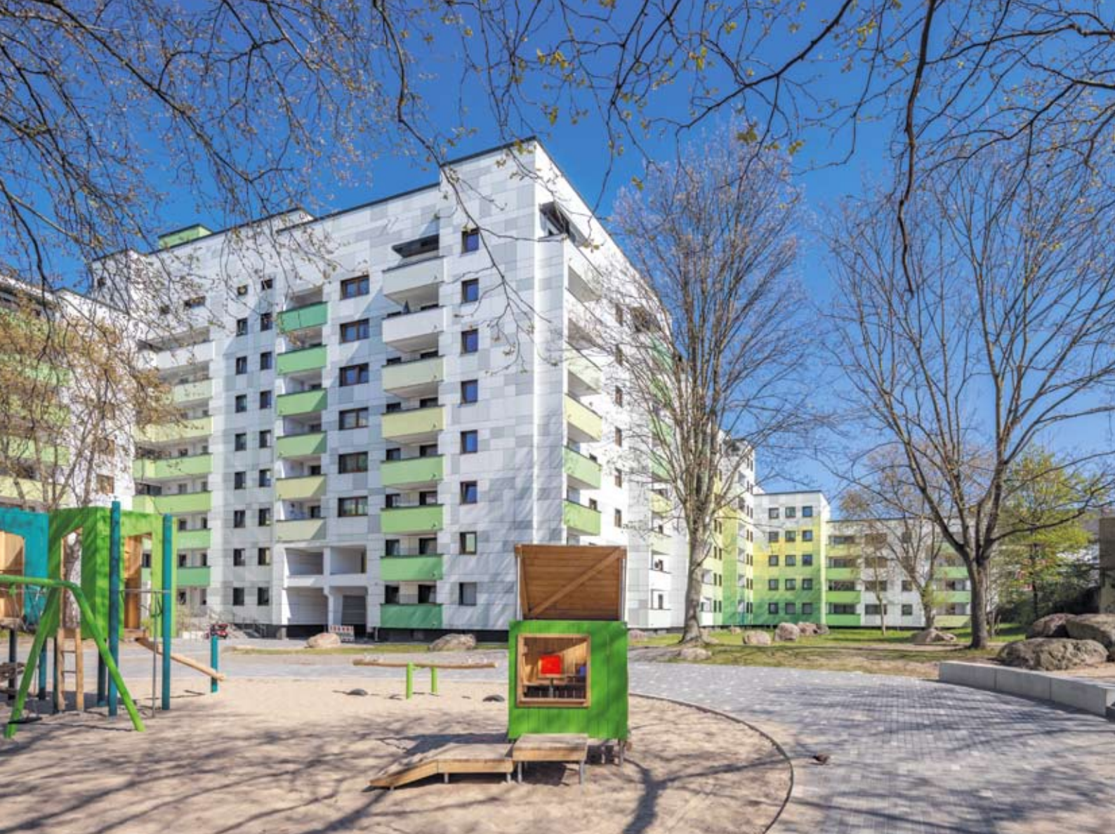
Fit for the future: the Citywohnpark in Duisburg with its identity-defining colour concept after renovation.
