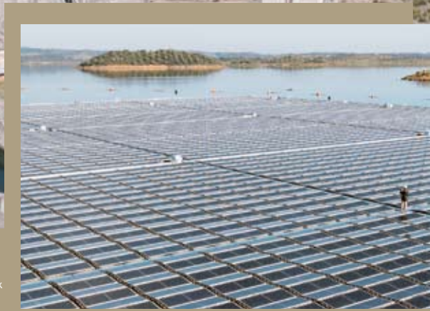
Photo above and photo right: A floating PV system with over 12,000 photovoltaic modules has been installed on the Alqueva reservoir in Portugal. It is equipped with a corrosion-resistant PVC cable management system that is suitable for outdoor use.
