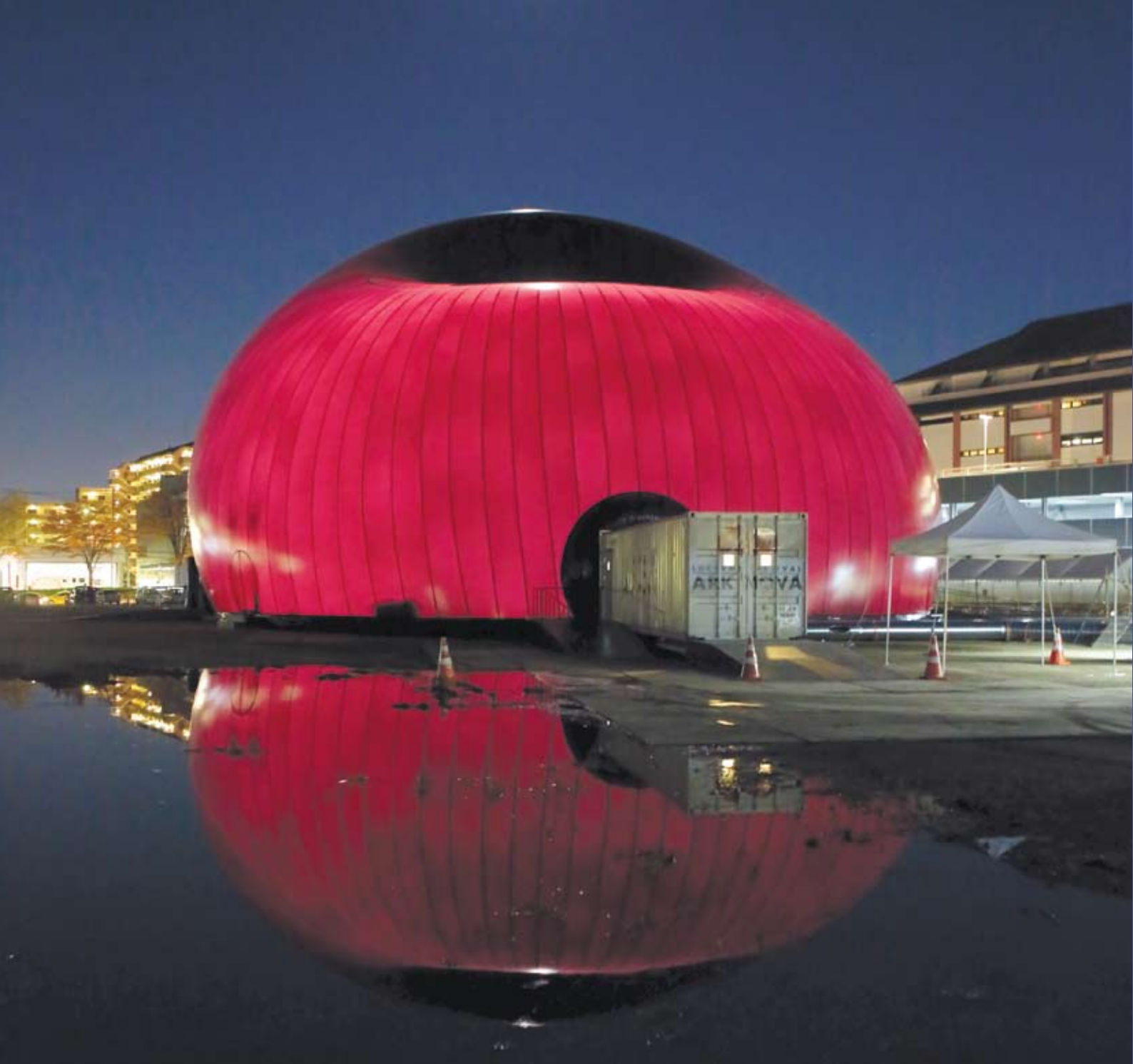
In 2014, the concert hall made of PVC-coated polyester was on display in Sendai, Japan.
